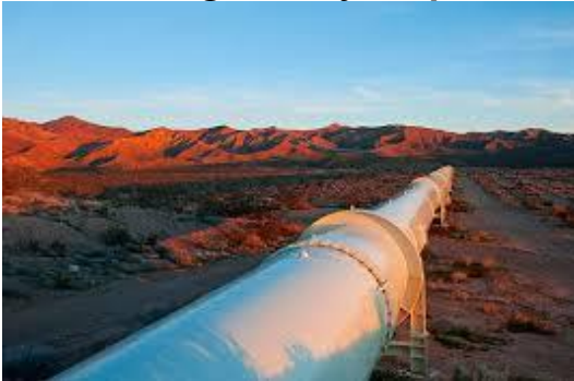
Communication Installation and Monitoring for Major Pipelines
